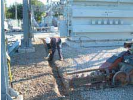
Above ground dike install for large facilities and equipment
