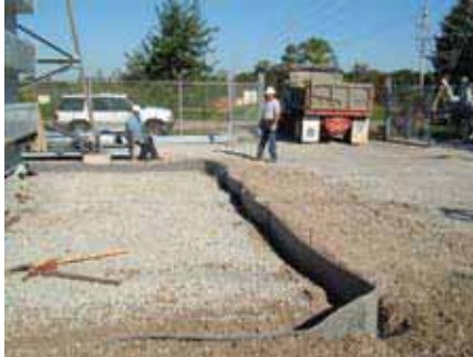
Above ground dike install for large facilities and equipment
