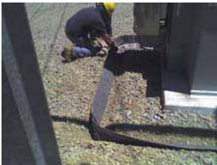
Above ground dike install for large facilities and equipment
